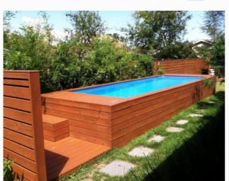
New Orleans-based architect Stefan Beese dove headfirst into recycled design by converting a defunct dumpster into a pristine backyard pool! The Pool Box is made from a 22' x 7' steel refuse container that has been lined with protective foam insulation and clad in pine wood slats. Best of all, the design's modular nature means that it can be easily packed up and transported to another location should the need arise.
