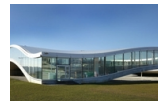
Built / Switzerland, Renens Rolux Learning Centre by SANAA (Sejima and Nishizawa and Associates) and Kazuyo Sejima & Associates
