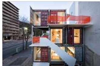
Shipping Container Workspaces
